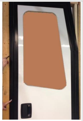
Place door into opening and mark/trace around perimeter with a pencil or other marking device. This is to show where frame needs to be when finished with install.
