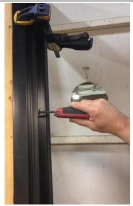
Tighten <u>all</u> socket head adjusting bolts until they are against sidewall and outside edge of outer frame is in line with mark/trace (done in first step).
