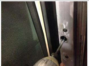
Fasten frame to sidewall by putting #10 screws (2" minimum length) through all the socket head adjusting bolts, into sidewall.
