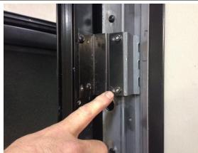
Screen door hinge has slotted mounting points on the hinge to allow adjustment and function of screen door. Adjust as needed.
