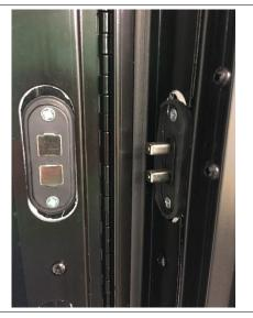
Contact plate to be wired for lock actuator ONLY.
