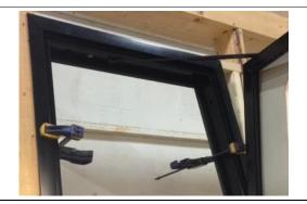
Open door and clamp top of outer frame (both sides) to wall.
