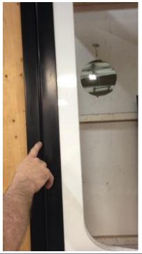
Close door. Check reveal between inner trim and outer frame, and open/close door to verify proper function of door. Reveal should be close to uniform all the way around the door. Adjust socket head screws and #10 screws as needed to obtain correct reveal and door function.
