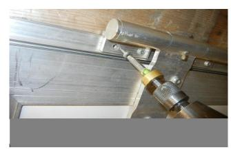
(2)-Drill through the hole where the screw has been taken from, using a drill and 5/16" drill bit.
