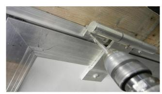
(3)-Place a 1/4" panhead bolt (third picture) through the hole from outside of door, and a t-nut(fourth picture) through the drilled hole from inside. Tighten securely. Repeat steps 1-3 until all hinge screws are replaced with bolts. Be careful not to remove more than 1 screw per hinge at a time or door may sag or become misaligned in outer frame.
